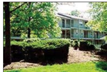
White Birch Crescent apartments on the east side of Franklin County.
