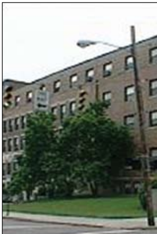
Bryden Road apartments in central Columbus.
